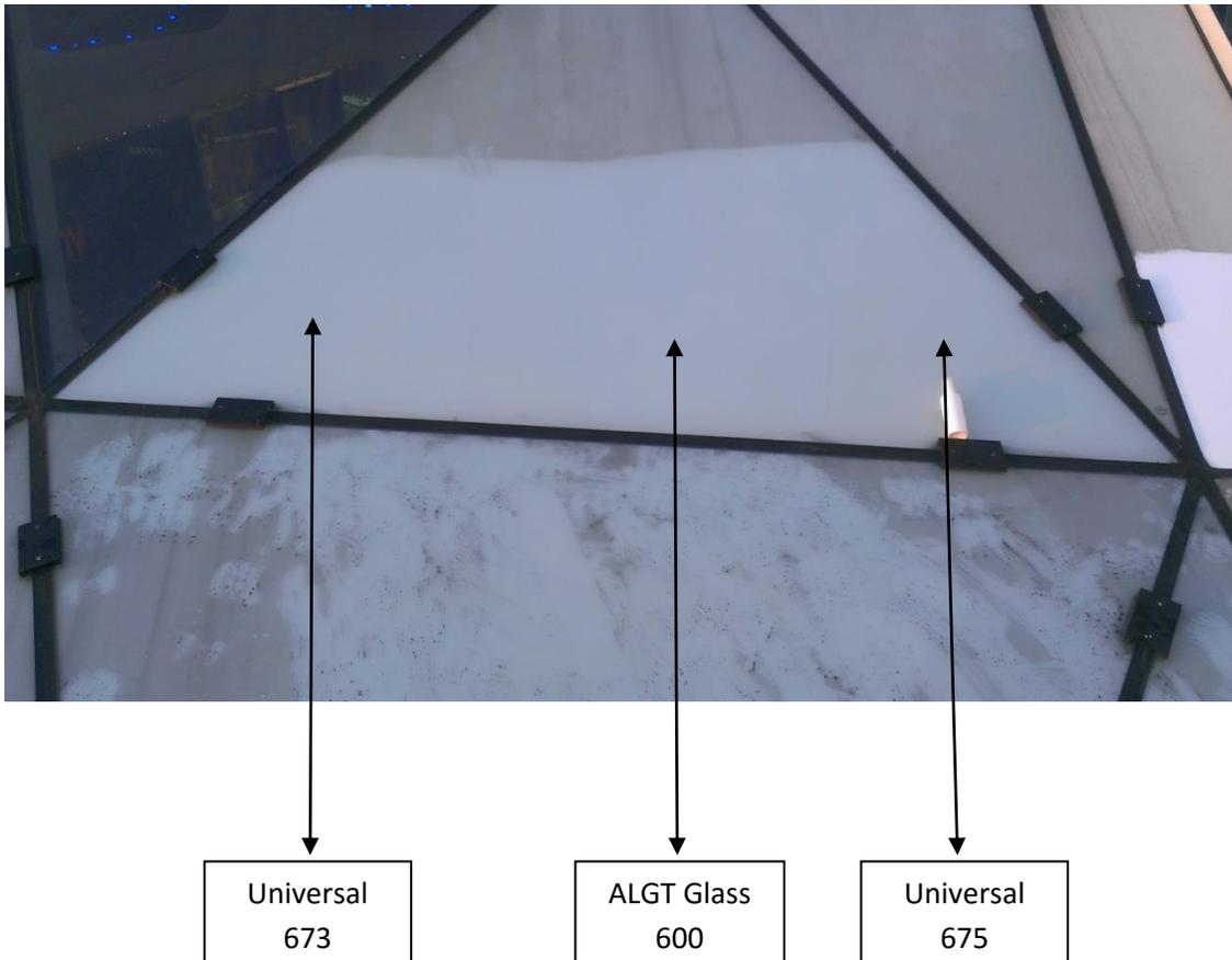
As noted, the surface of the glass was heavily contaminated. Cleaning with IPA showed that after 10 cleaning actions the glass was still contaminated as the soiling was ingrained.
