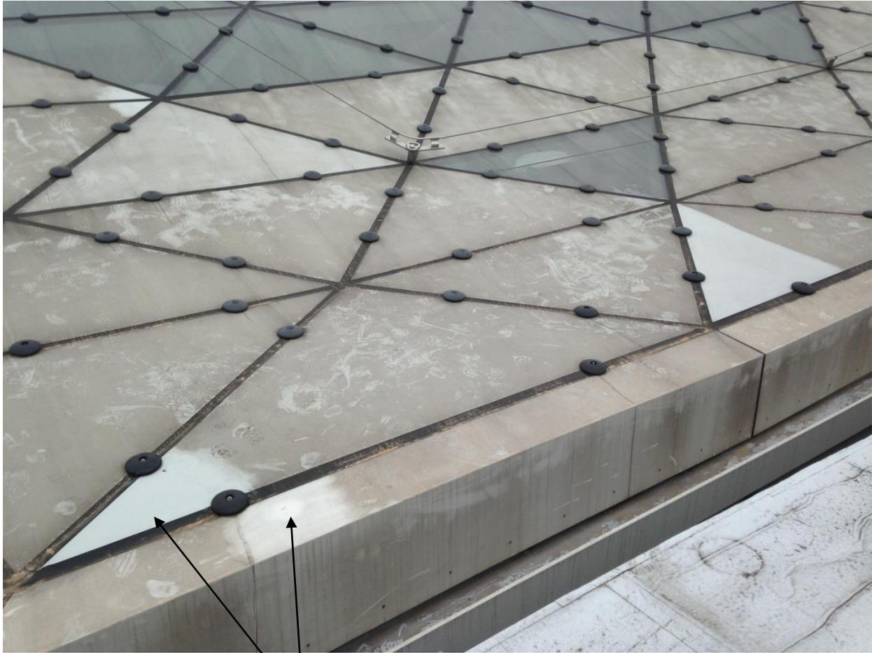
Acrylic area cleaned with stainless steel cleaner BLU1000. Note that it is brighter than the area cleaned with Biosativa® as the soiling is ingrained within the surface. Cleaning with this process creates an “as new” appearance but it will require more cleaning effort in the first instance.
