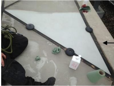
This area is a mixture of glass and acrylic panels. The acrylic panels are heavily soiled and require additional cleaning. Biosativa® cleans the area quite effectively as noted in the images, but cleaning the plastic/acrylic surface with stainless steel cleaner BLU1000 is probably required in order to provide a surface suitable for coating
