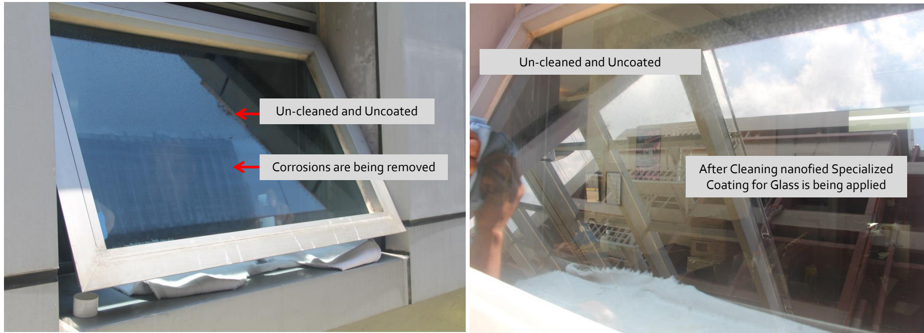
DMCI Building Glass window cleaned and protected with nanofied Specialized Coating for Glass
