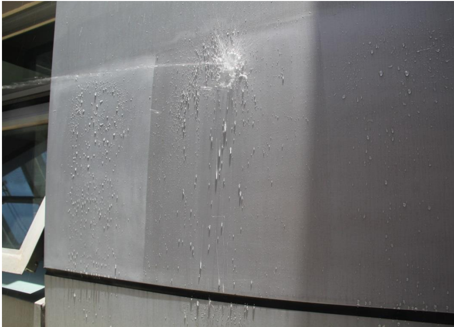
Coated aluminum cladding remains clean and without corrosion after 1 week, water is sprayed on aluminum cladding notice that water beads and is being repelled by the coating
