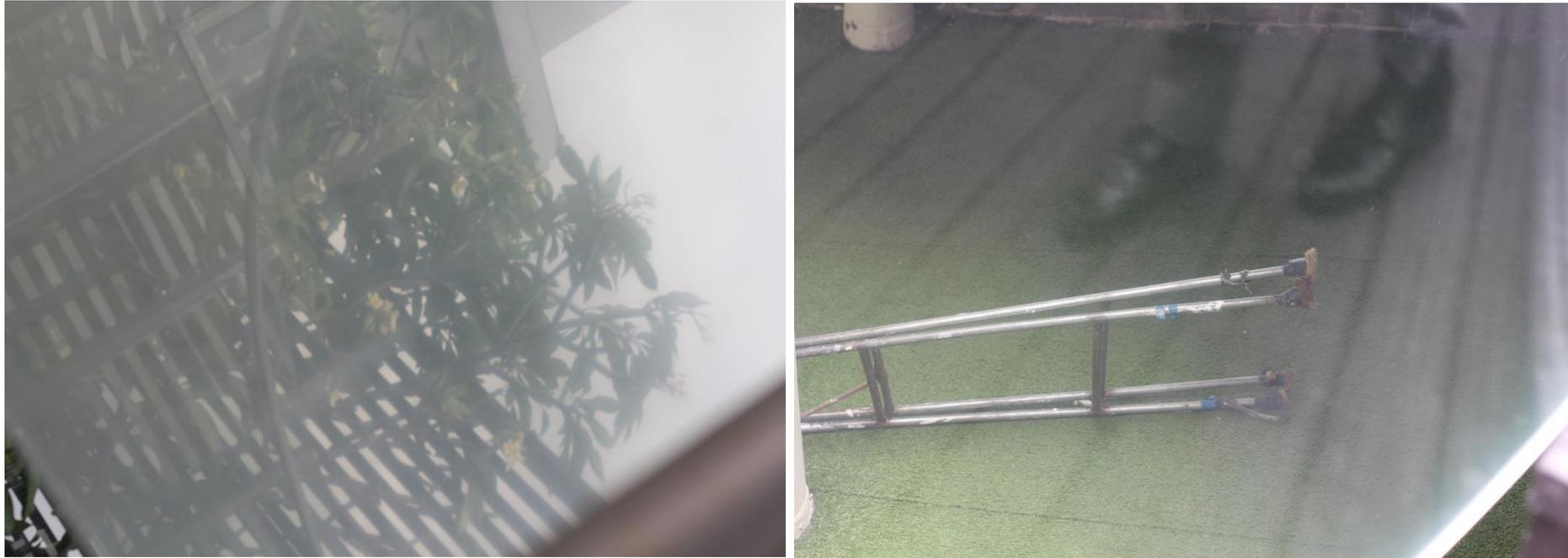
Visible glass corrosions from chemical residue, acid rain, pollution and bird droppings. When it dries and hardens it becomes very hard, sometimes impossible to remove.
