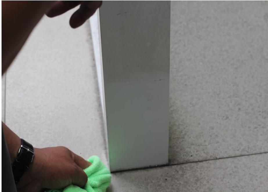
Corrosion and Dirt is removed from Powder Coated Panels using nanofied special cleaner.
