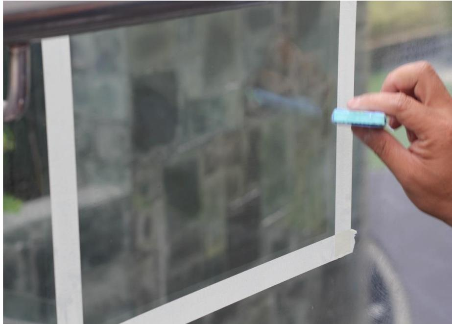
After cleaning nanofied specialized coating for glass is being applied to protect cleaned glass panel from corrosions.
