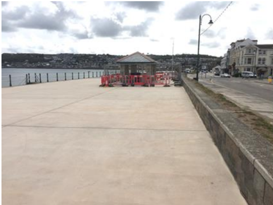
after pressure washing
