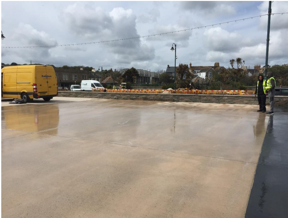
The area was cleaned with a pressure washer
