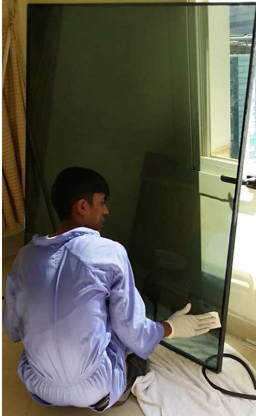
Application of ALGT Glass Coating 7601
