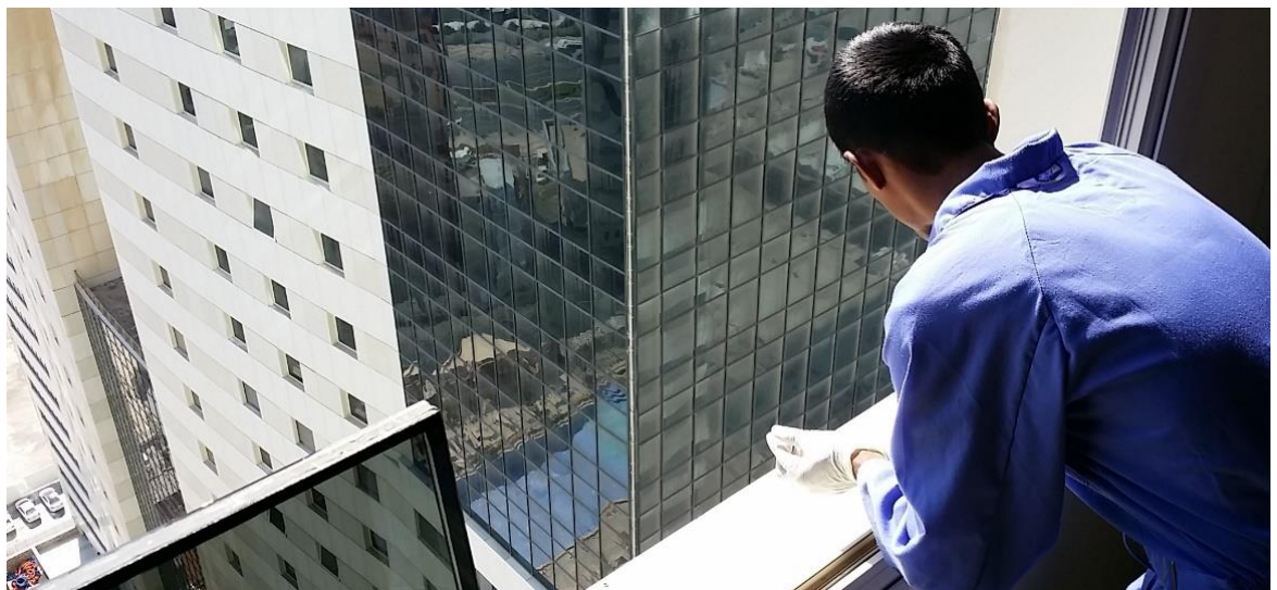
Coating the windowsill with ALGT Permanent Protector 640
