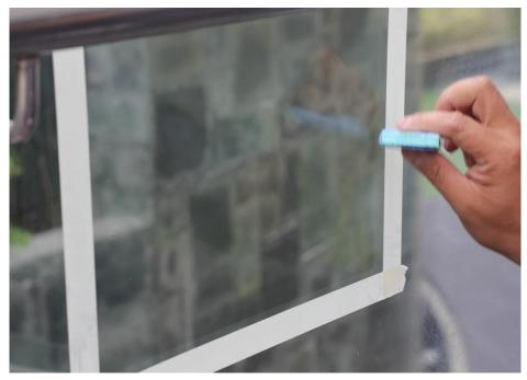
After cleaning nanofied specialized coating for glass is being applied to protect cleaned glass panel from corrosions.
