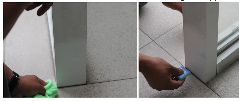
Corrosion and Dirt is removed from Powder Coated Panels using nanofied special cleaner.
