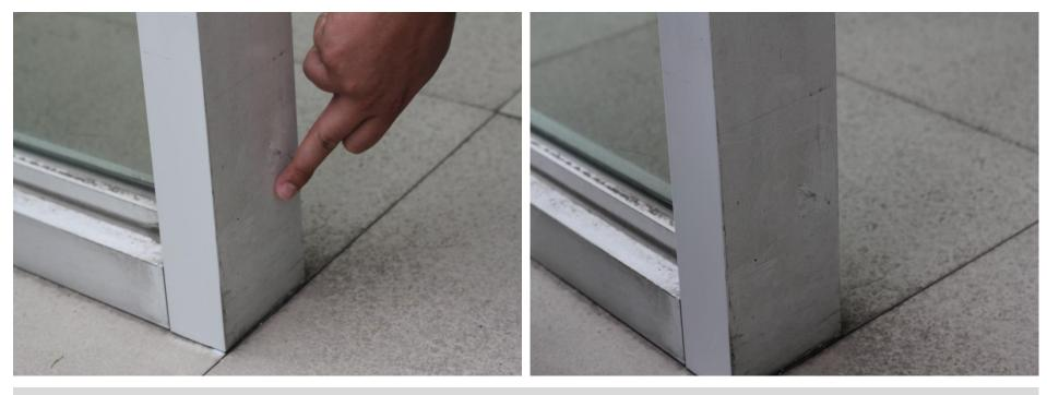
Un-cleaned and Unprotected Powder Coated window and Door panels. Powder Coated panels are very hard to maintain and protect specially outdoors. Cleaning and Maintaining Powder Coated Panels are very time consuming and expensive.
