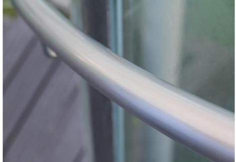
After 3 weeks, cleaned and protected stainless handrail is corrosion free and easy to clean.
