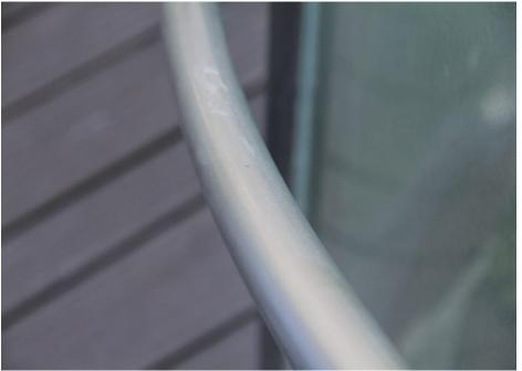
Unprotected stainless hand rail shows corrosion like white rust, watermarks and grime on stainless handrail. Corrosion on stainless steel is very hard to remove sometimes may cause permanent damage to stainless steel
