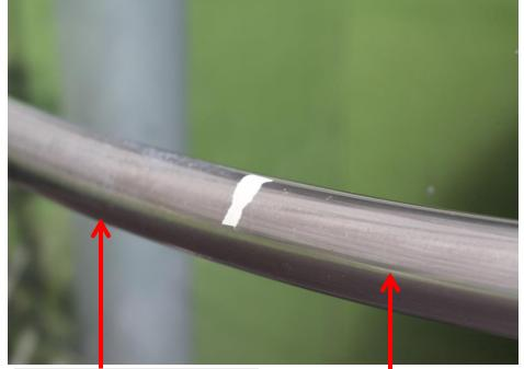
Un-cleaned and Unprotected stainless hand rail. White rust, watermarks and grimes is very visible
