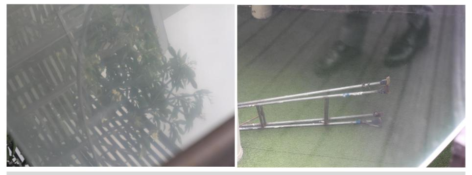
Visible glass corrosions from chemical residue, acid rain, pollution and bird droppings. When it dries and hardens it becomes very hard, sometimes impossible to remove.
