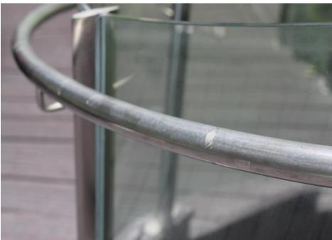
Un-cleaned and Unprotected stainless hand rail. Corrosion like white rust, watermarks and grime on stainless handrail is very visible. Corrosion on stainless steel is very hard to remove sometimes may cause permanent damage to stainless steel
