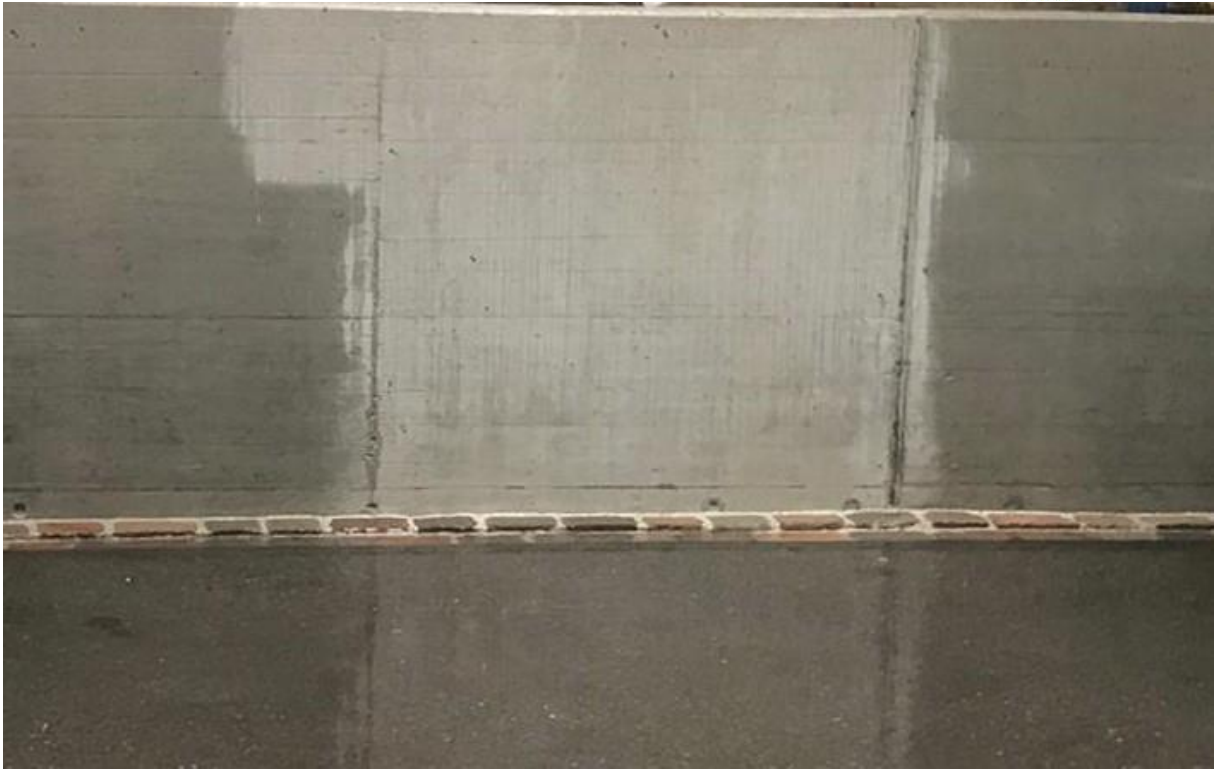
coated side during rain
