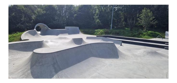
The newly cleaned surface not only looks like new but cleaning with Biosativa® has resulted in the removal of oils and sugars, (from soft drinks). These contaminants must be removed in order to allow for optimum bonding conditions for the application of the protective layer.
