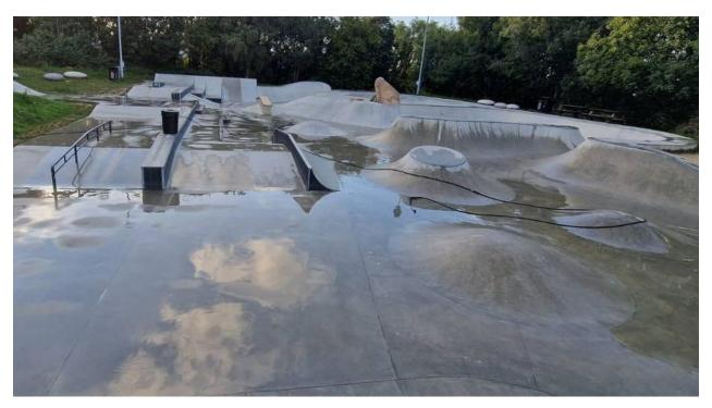
Biosativa was spray applied at 1:20. The surface was then rinsed with a "light" pressure washer.
