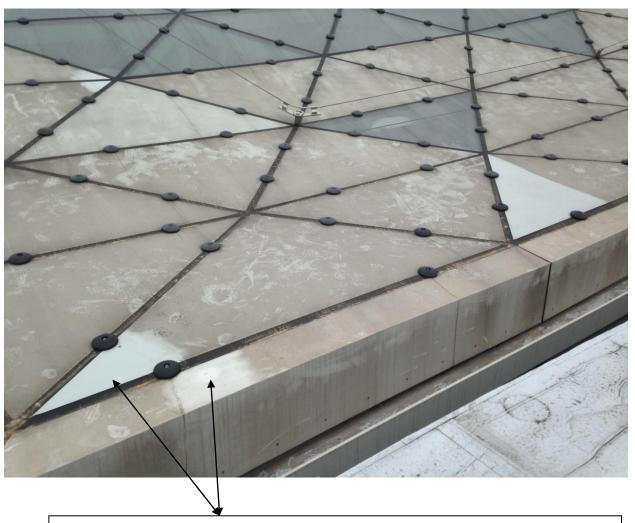
Acrylic area cleaned with stainless steel cleaner BLU1000. Note that it is brighter than the area cleaned with Biosativa® as the soiling is ingrained within the surface. Cleaning with this process creates an "as new" appearance but it will require more cleaning effort in the first instance.
