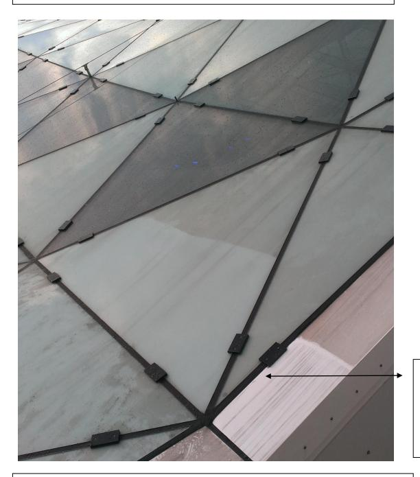
This area is completely clean as it has not been exposed to "run off"
